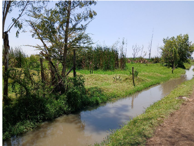
Figure 35: Trench dug by the County Government in Kapuothe to redirect overflow from River Wigwa
