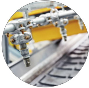
Fire extinguishing system
