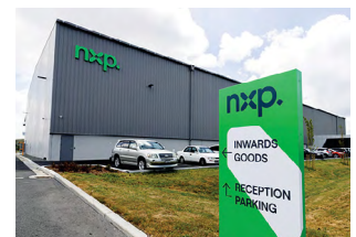
NXP Christchurch 11 Gallagher Drive, Hornby South, 8042
