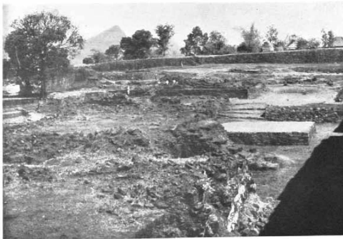
Pachad, Jijamata palace: A, before and B, after repairs. See p. 146
