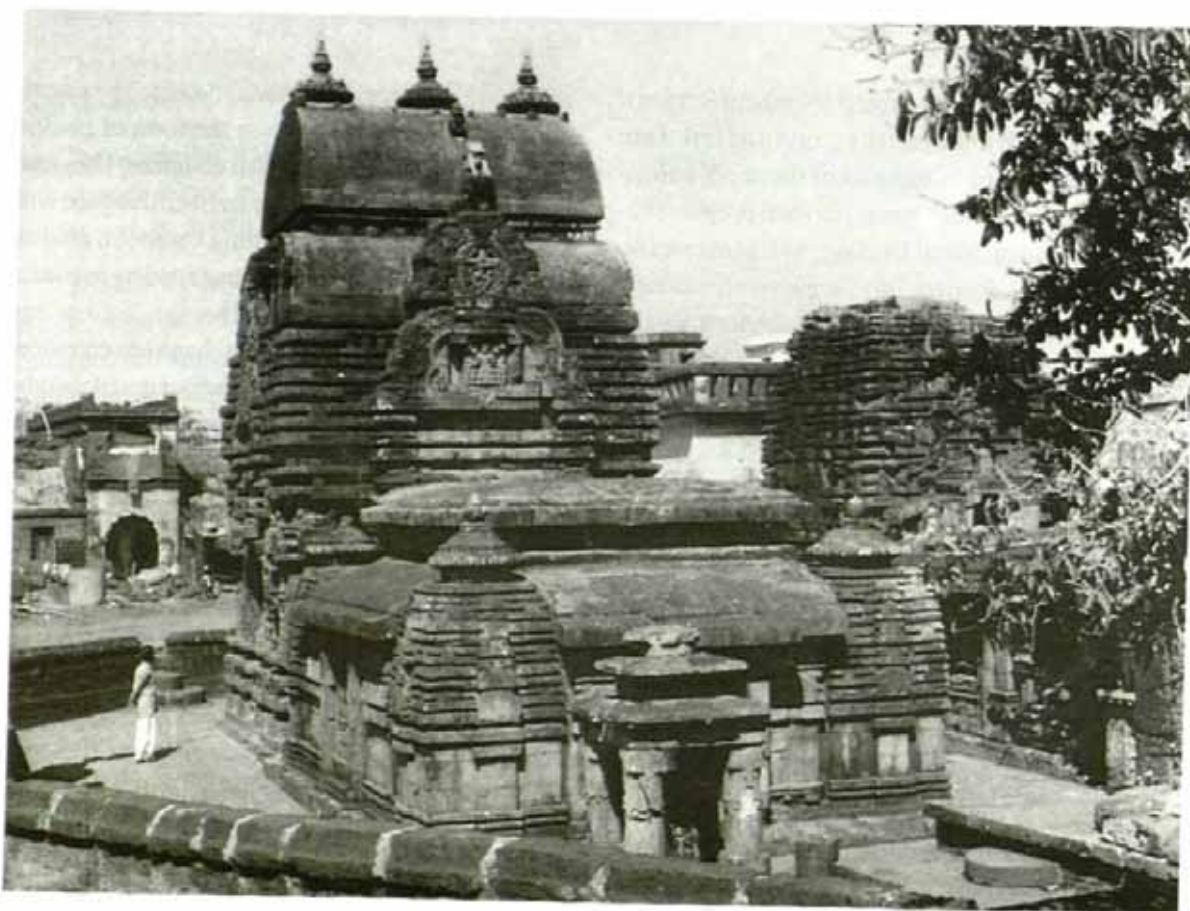
Bhubaneswar, Vaital Deul : general view showing khakharamastaka
