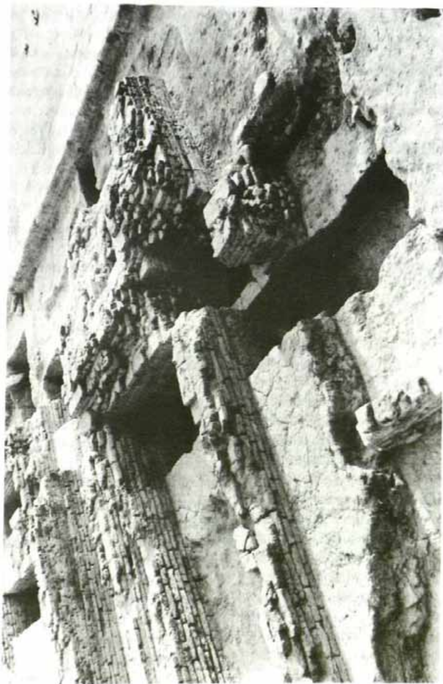
Paithan : different structural phases of northern building
