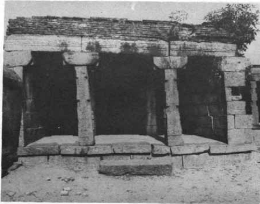
150 Venkatesa Perumal temple, Tirumukkudal : View showing before the removal and re-erection of Anjaneya subshrine before conservation. See page 225
