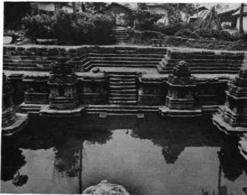
115 Hulikera : View showing the western wing of Kalyani after conservation. See page 214
