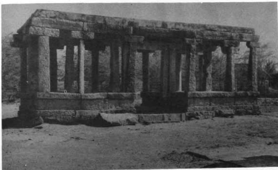
142 Kilputtur Svyabhunatha Temple : General view of the Mandapa before conservation. See page 224
