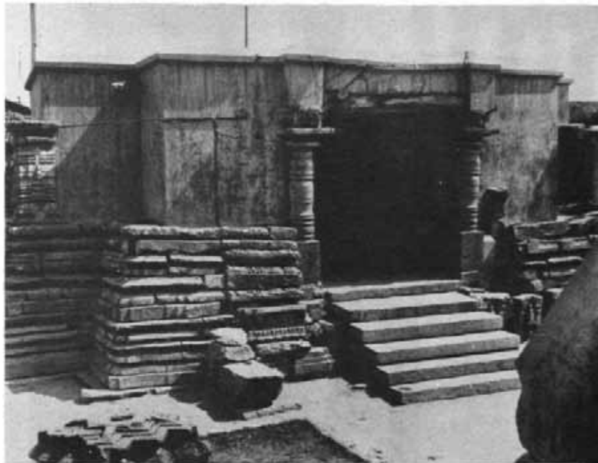
116 Basral : General view of the entrance Mandapa of Malikarjuna temple before conservation. See page 215
