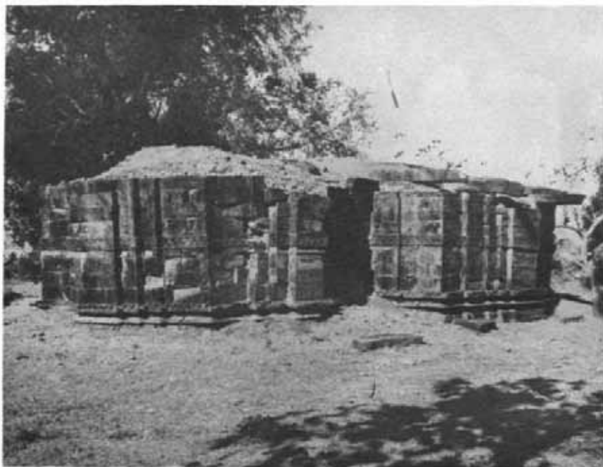
118 Bandalike Anekal sameswar temple : View showing the southern side of the temple before conservation. See page 215
