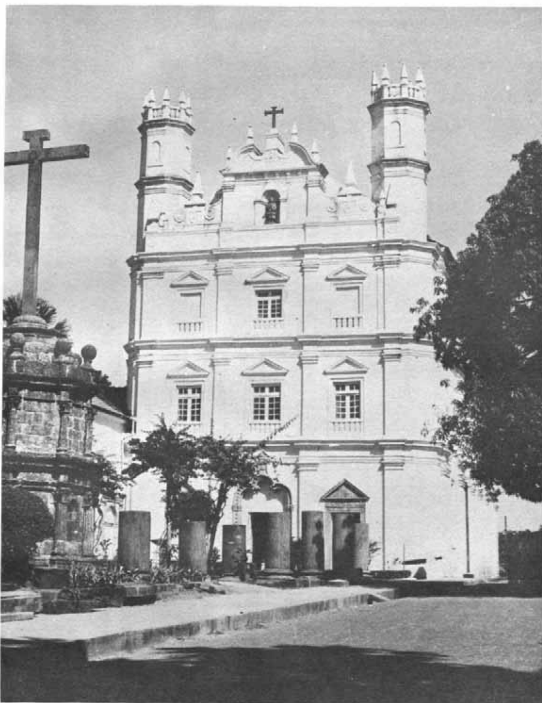
157 St. Assisi Church : General view of the facade from west after conservation. See page 227
