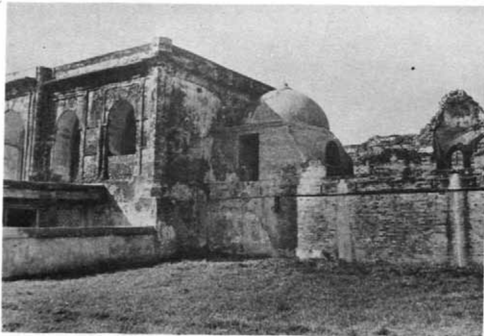
111 Katra : Dome of Katra mosque of east after conservation. See page 210
