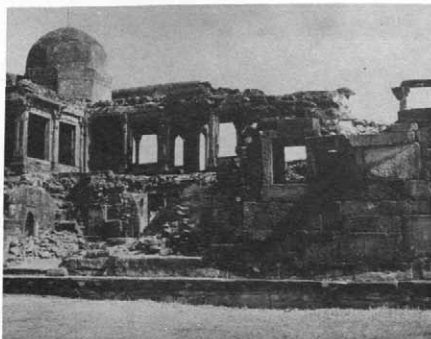
102 Raisen Fort : Close-up view of Jinjhari Mahal before conservation. See page 207
