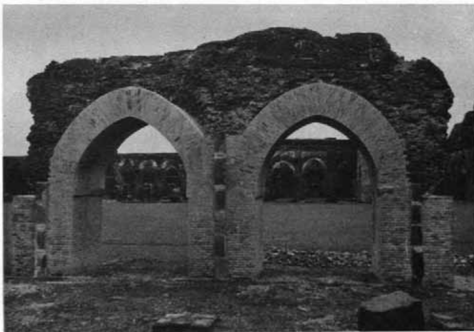
109 Adina : Two arches inside Adina Mosque in east after conservation. See page 210
