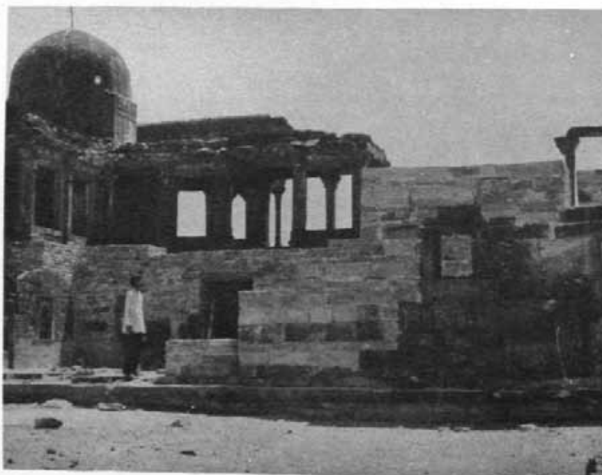
103 Raisen Fort : Close-up view of Jinjhari Mahal after conservation. See page 207
