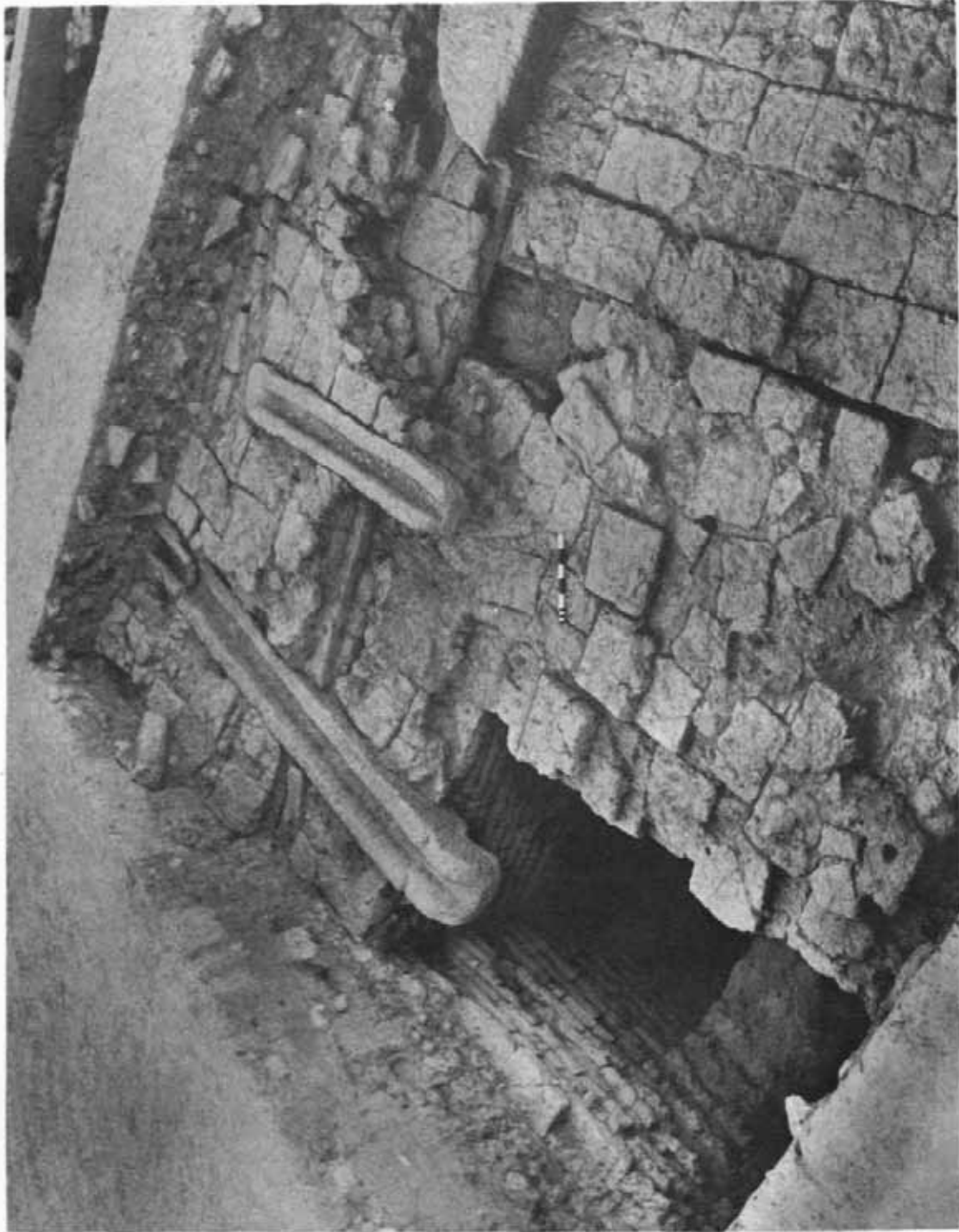
18 Goraj (Mahadeopura): Partly exposed brick structure with stone drains ( Pranals ) and Kunda . See page 23
