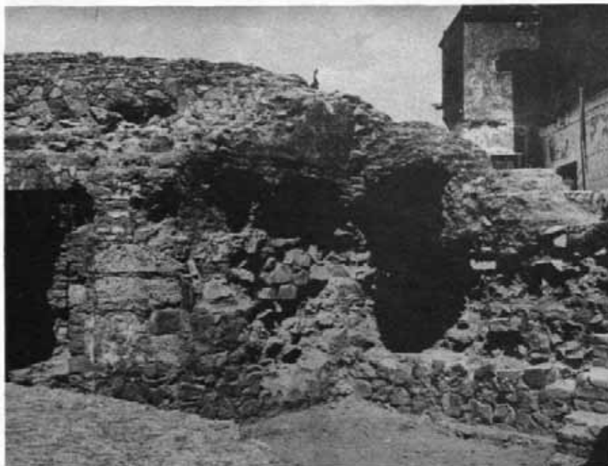
98 Burhanpur : Close-up view of Hammam before conservation. See page 206
