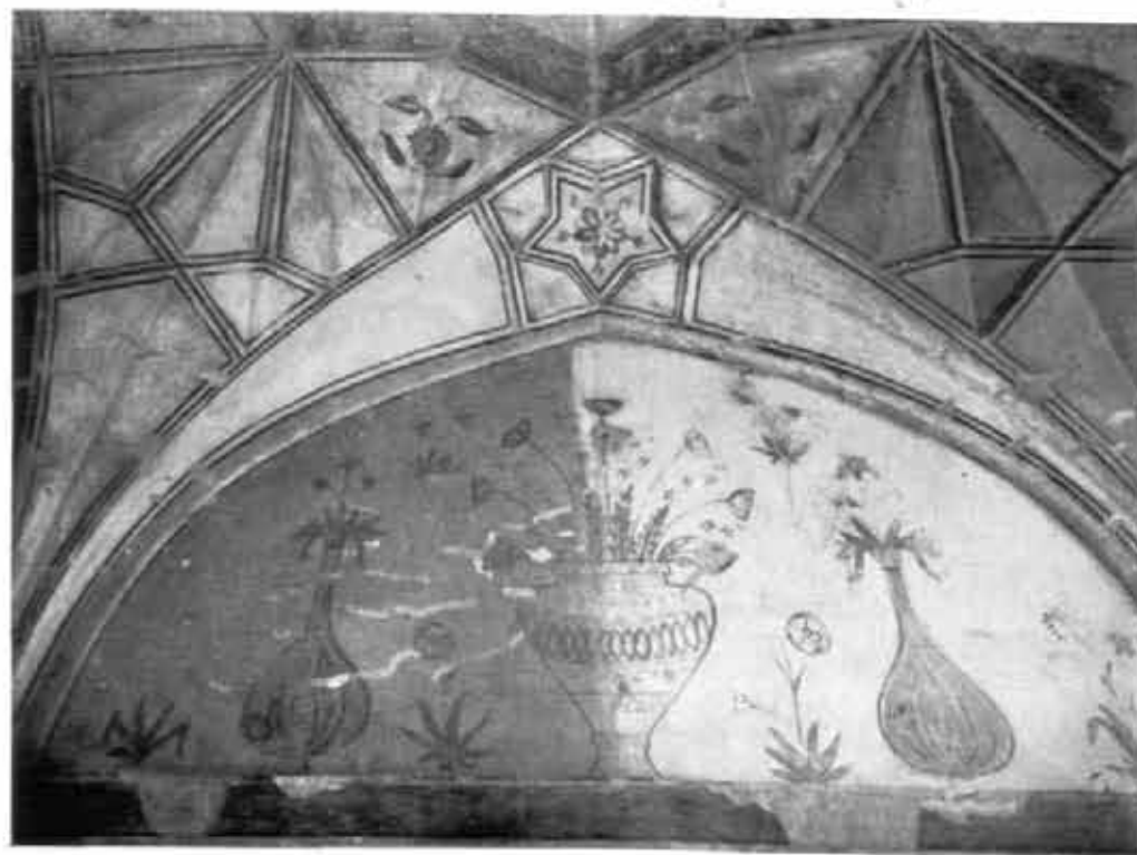
B. Allahabad : Khusro-bagh, painting during treatment. See page 110
