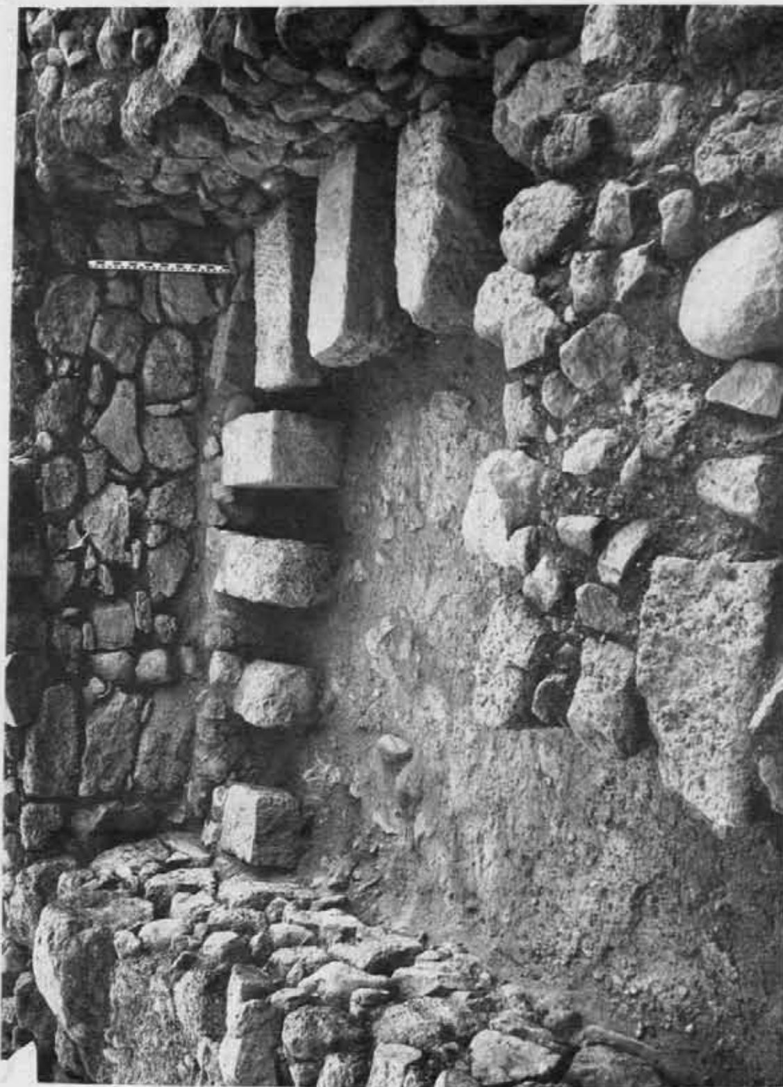
Daulatabad : exposed toilets. See p. 83
