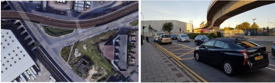
Figure 7: A112 Connaught Rd / Hartmann Rd Junction
