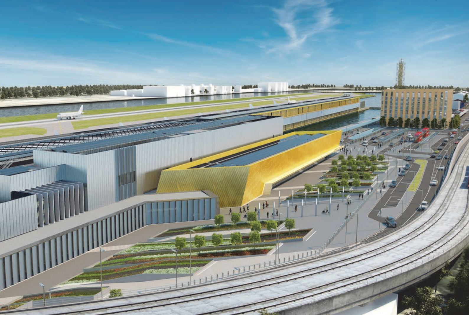
CADP looking north east
