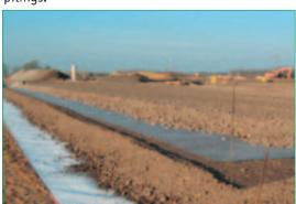
About 7,000 m² of Combigrid® 60/60 Q1 251 GRK 4 were used as the bottom reinforcement layer. Combigrid® ensured the separation and filtration between the embankment's bulk material and the finely grained subsoil along with providing the first layer of soil reinforcement.
