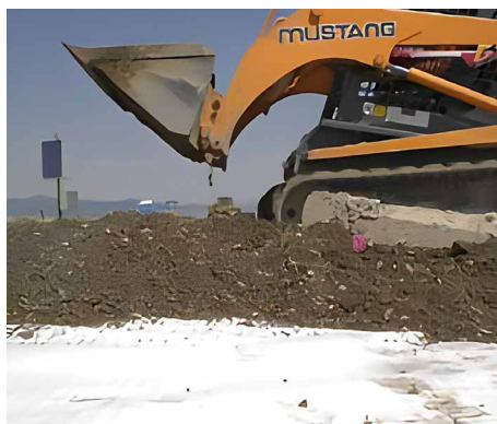
Fig. 11 Base course aggregate installed over Combigrd® for improved roadway performance.
