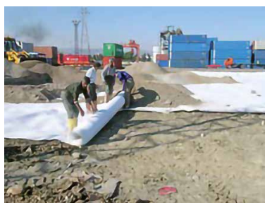
Fig. 13 Unrolling and overlapping of Combigrig® over a soft subgrade.
