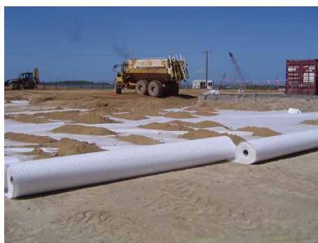
Fig. 3 Combigrig® installed as base course reinforcement where multi-directional stiffness is of great importance.
