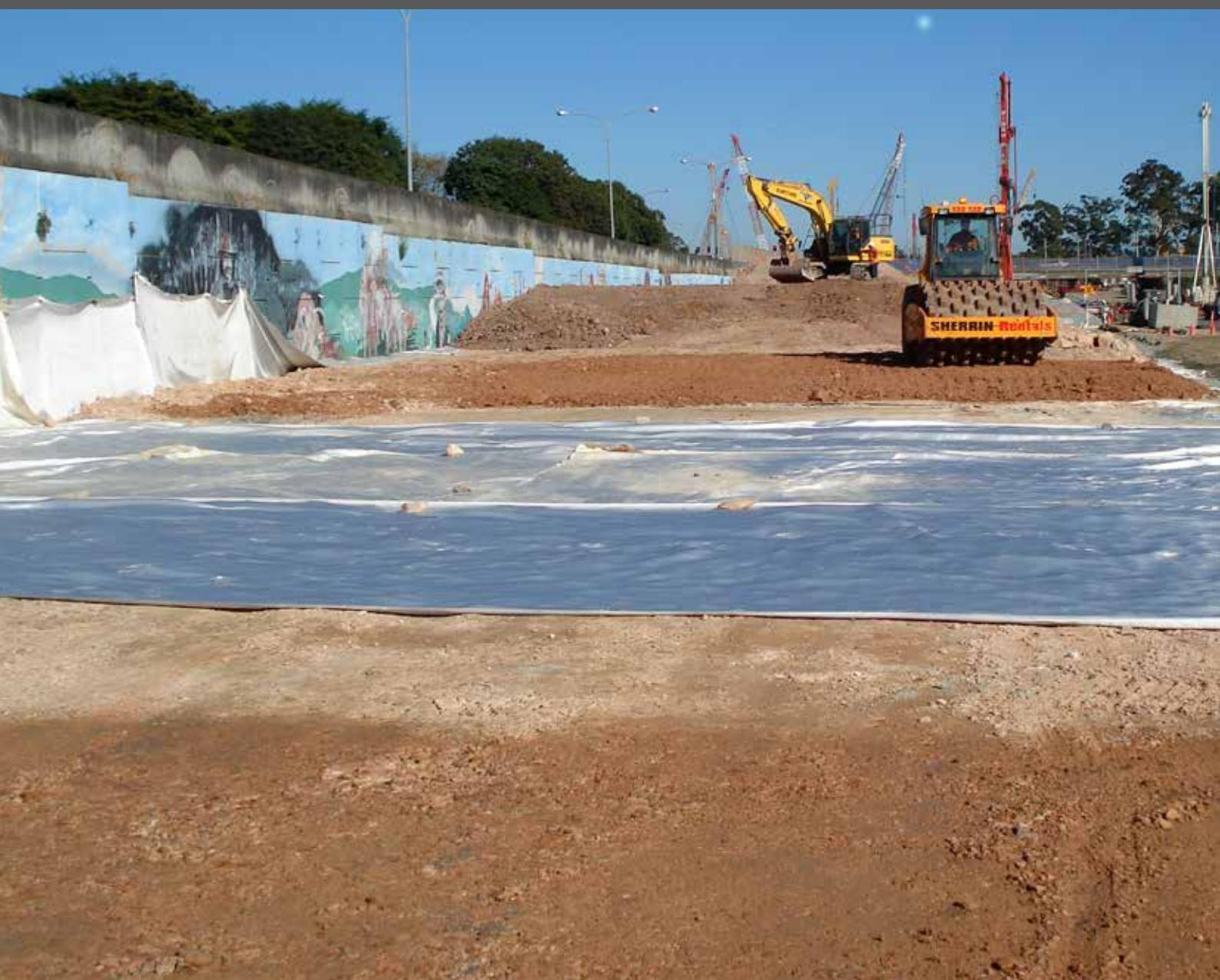
Global Synthetics provide the ACETex® structural geotextile, a product option that offers design engineers a cost effective and proven alternative to many traditional ground treatment options.
