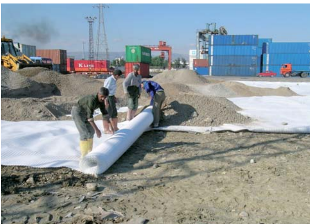
Fig. 13 Unrolling and overlapping of Combigrid® over a soft subgrade
