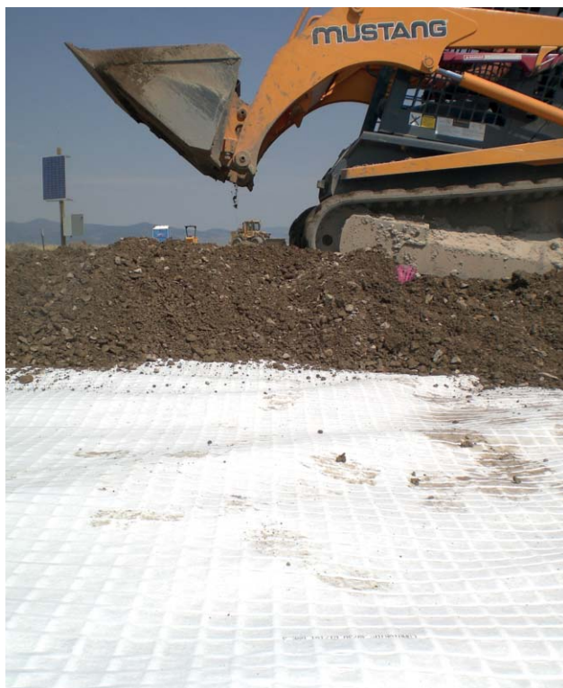
Fig. 11 Base course aggregate installed over Combigrid® for improved roadway performance
