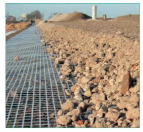
Fig. 19 Crushed base course material over Secugrid® for base stabilisation in access roads
