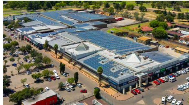
Kriel Mall - Checkers extension for 5 additional years- GLA 3 142 m 2 . Dischem expansion completed
