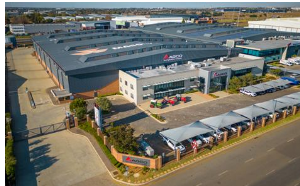
Completed solar installations at 16 Pama
