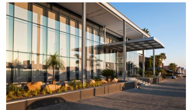
Completed solar installation at 130 Gazelle
