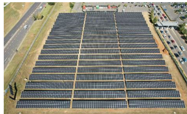
Solar farm completed at Newcastle Mall
