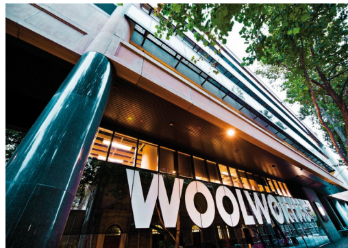
Early Renewal for further 6 years at Woolworths house f(30,400m 2 )
