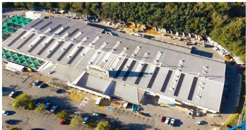
Solar installation: Builders Warehouse Zambezi, Montana, Gauteng GLA: 8 908 m 2
