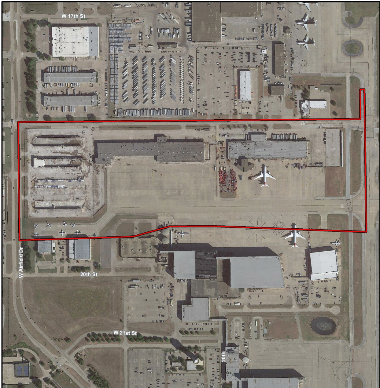
Figure 1 19th Street Cargo Redevelopment Project Site west side of DFW
