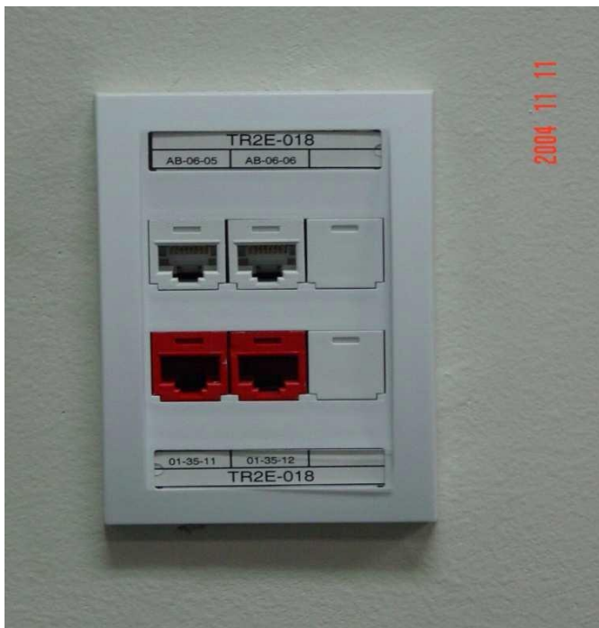
Figure 2 – Wall Area Outlet Faceplate Labeling.
