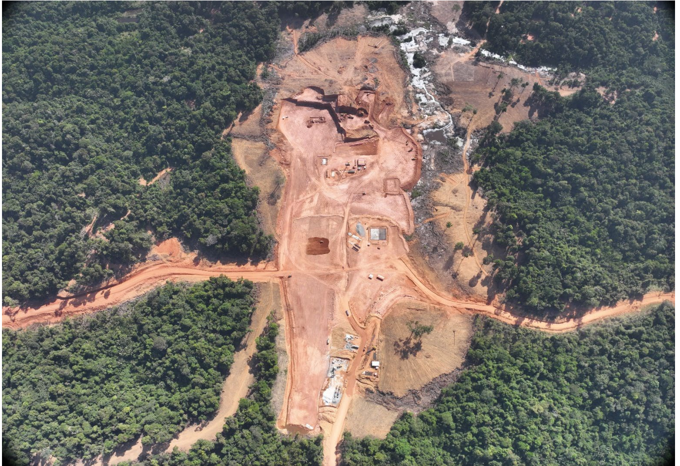
Figure 1 - Earthwork Progress at Industrial Area
