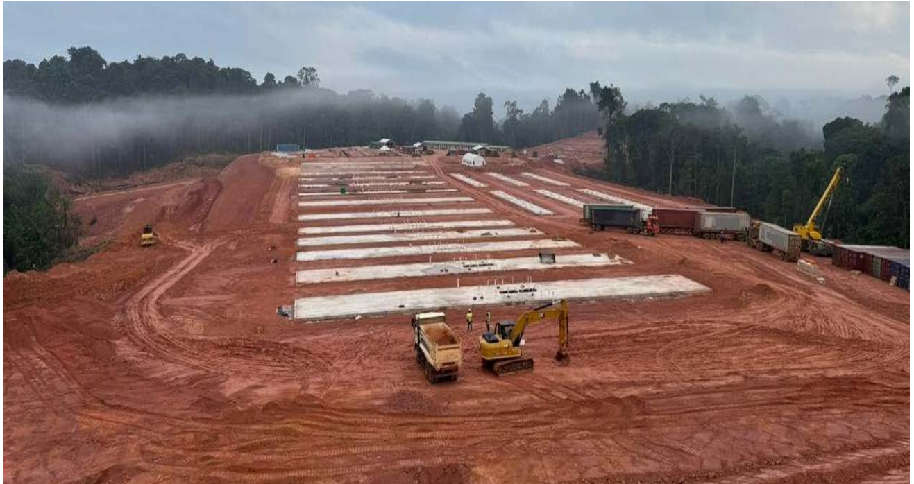
Figure 2 – Permanent Camp Construction
