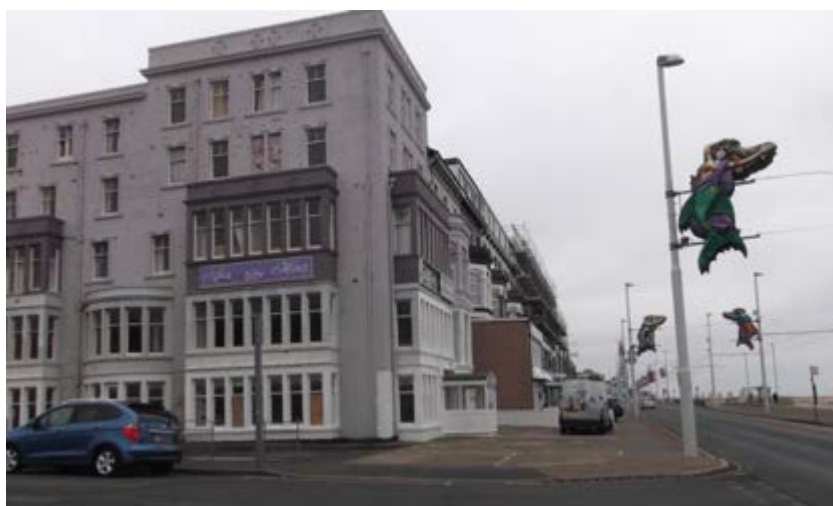
Figure 5: A dilapidated B&B in central Blackpool
