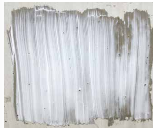
Iso-Tek™ 8501 Gel applied to a 14,000 PSI vertical wall on 432 Park Ave, NYC.
