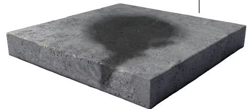
Untreated Concrete, Showing Water, Salt And Stain Intrusion
