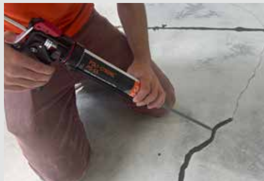
CRACK FILLER SEAL AND SMOOTH OUT IMPERFECTIONS
