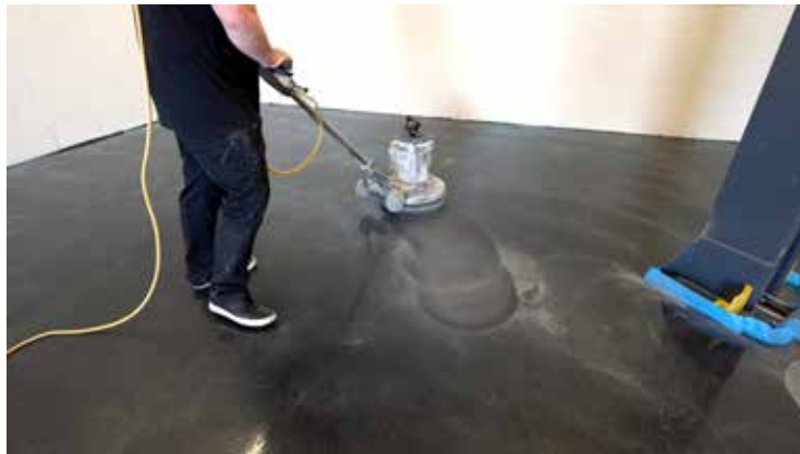
SAND - 80/100 GRIT SCREEN REDUCES SURFACE TENSION - IMPROVES ADHESION
