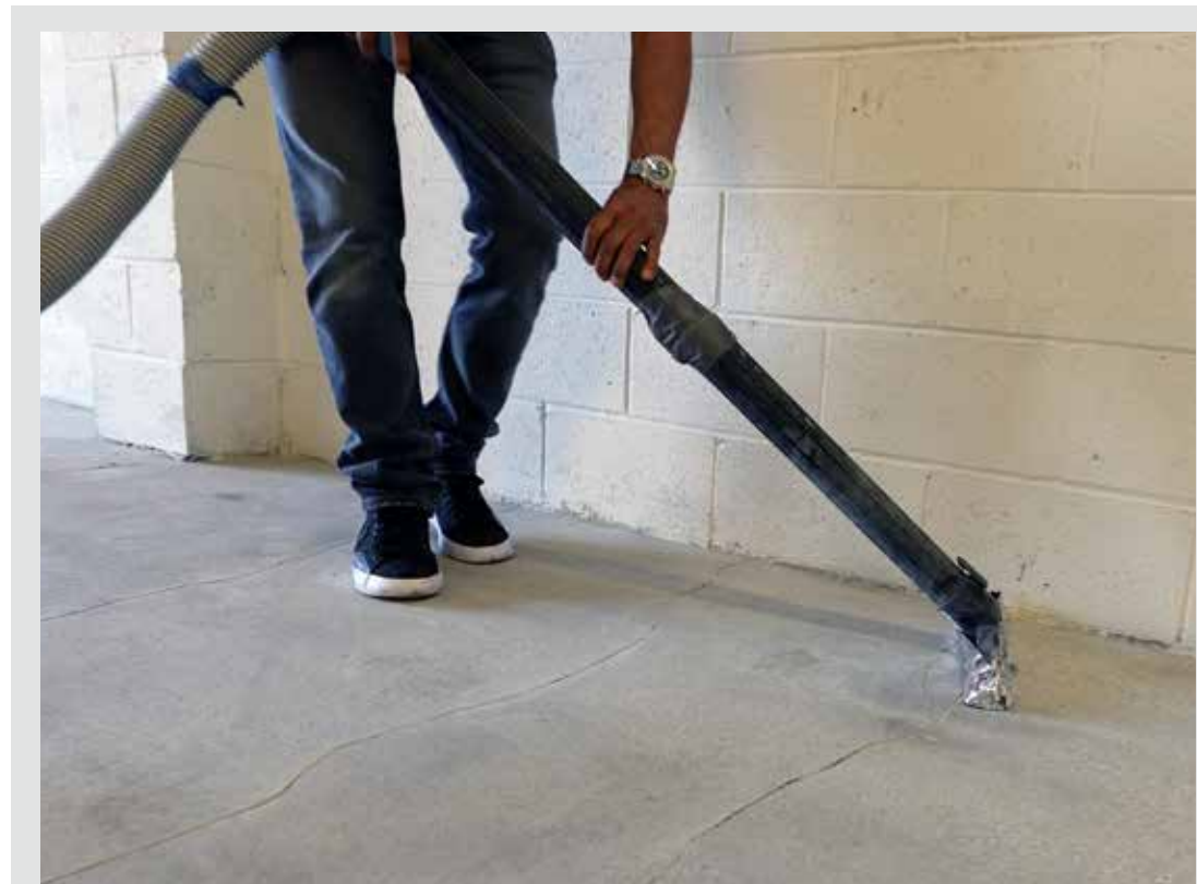
VACUUM ENTIRE FLOOR REMOVE ALL SURFACE DUST AND DEBRIS
