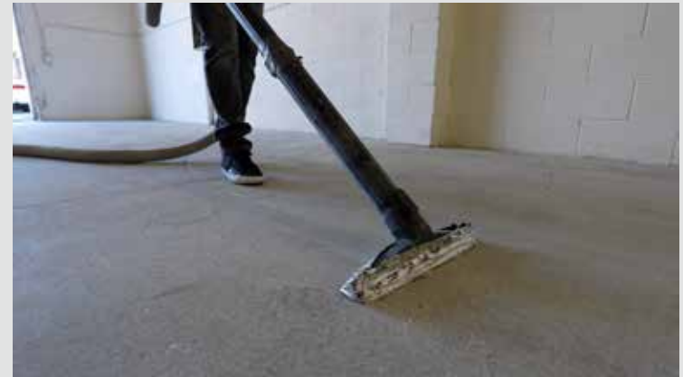
VACUUM ENTIRE FLOOR REMOVE ALL DUST & DEBRIS
