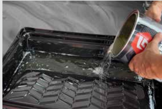
POUR INTO PAINT TRAY DIP / ROLL PROCESS SIMILAR TO PAINT
