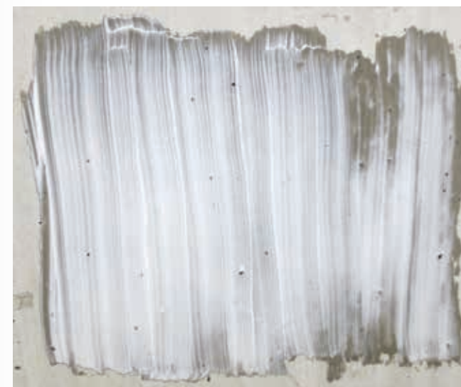
Iso-Tek™ 8501 Gel applied to a 14,000 PSI vertical wall on 432 Park Ave, NYC.
