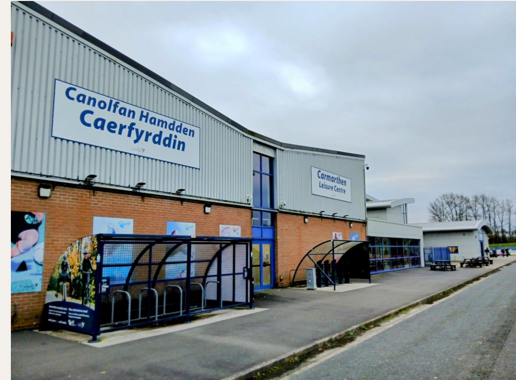
Image: Carmarthen Leisure Centre
