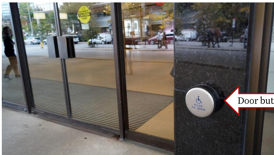
This picture shows the automated door and push-to-open button for our building.
