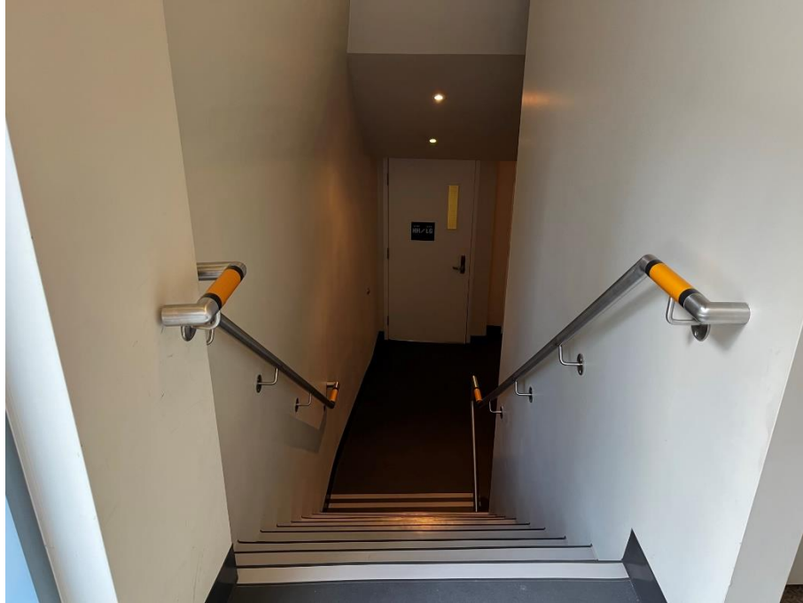
This picture shows the set of stairs leading down to the B1 level from the Yonge Street entrance.
