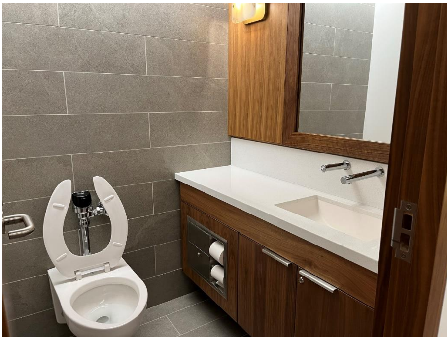
This picture shows one of the gender-neutral washrooms on the west side of the main lobby.
