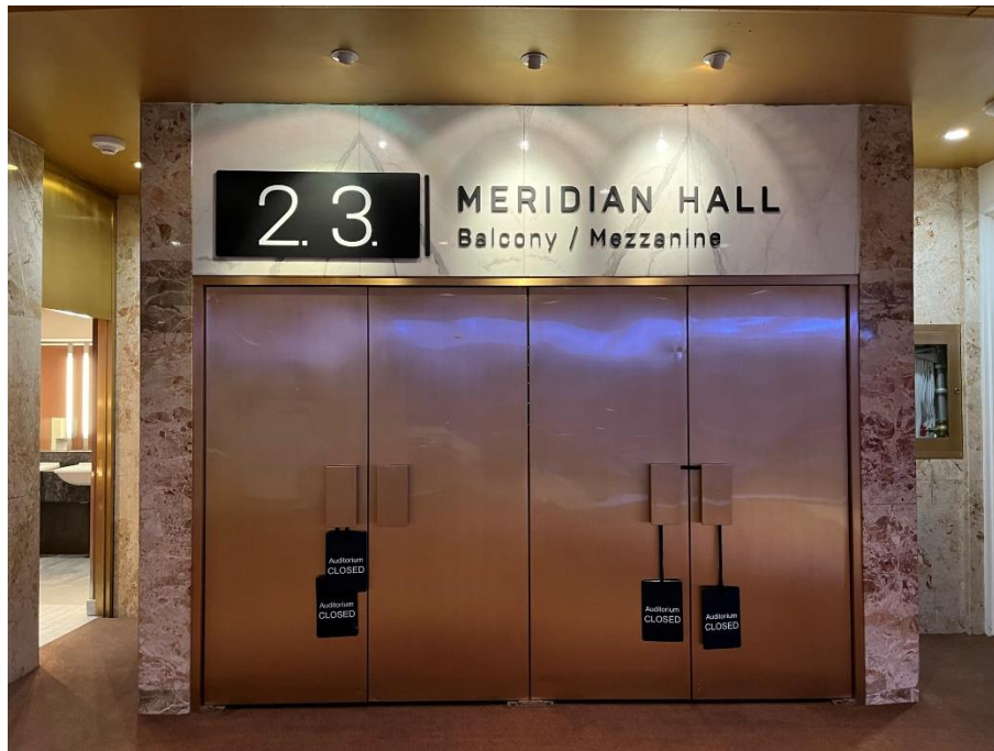
This picture shows the set of doors for aisles 2 to 3 into the auditorium from the mezzanine.
