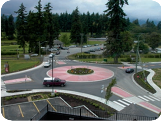
A modern roundabout at Chemainus Road and Henry Road, North Cowichan
