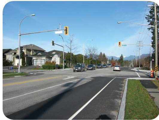
84th Avenue and 168th Street, Surrey New traffic signal, and left turn lanes
