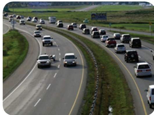
Median Cable Barrier – Highway 1 near Chilliwack
