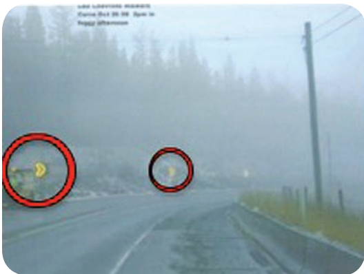
LED chevron signs lit during fog
