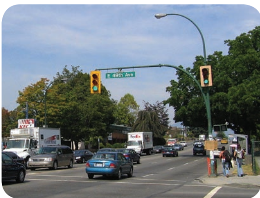
Tertiary signal head shown on the right hand side
