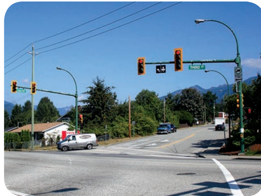
300mm signal lenses improve the visibility of traffic signals
