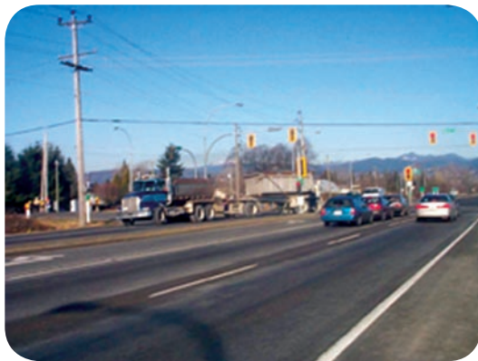
Road Safety Audit – Highway 1 – Clayburn Road to Harris Road
