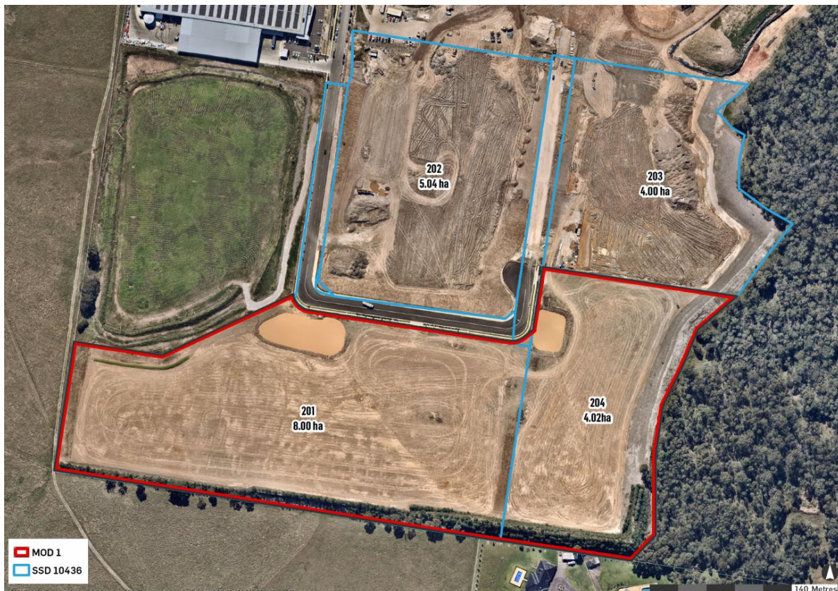
Figure 1 Aerial photograph of the site
