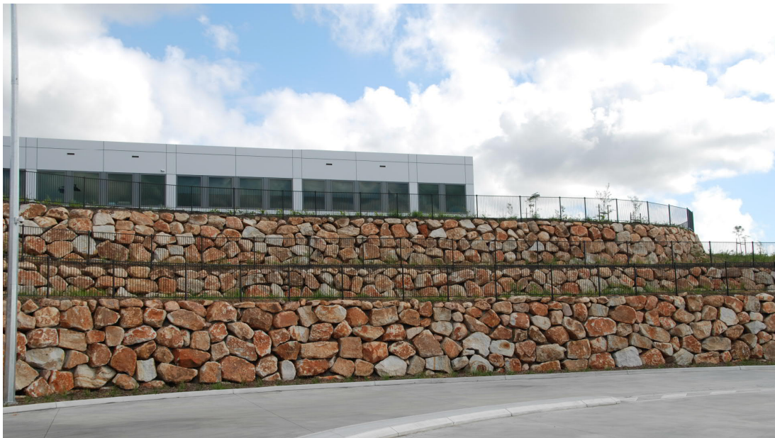
Figure 8: Tiered boulder retaining wall
