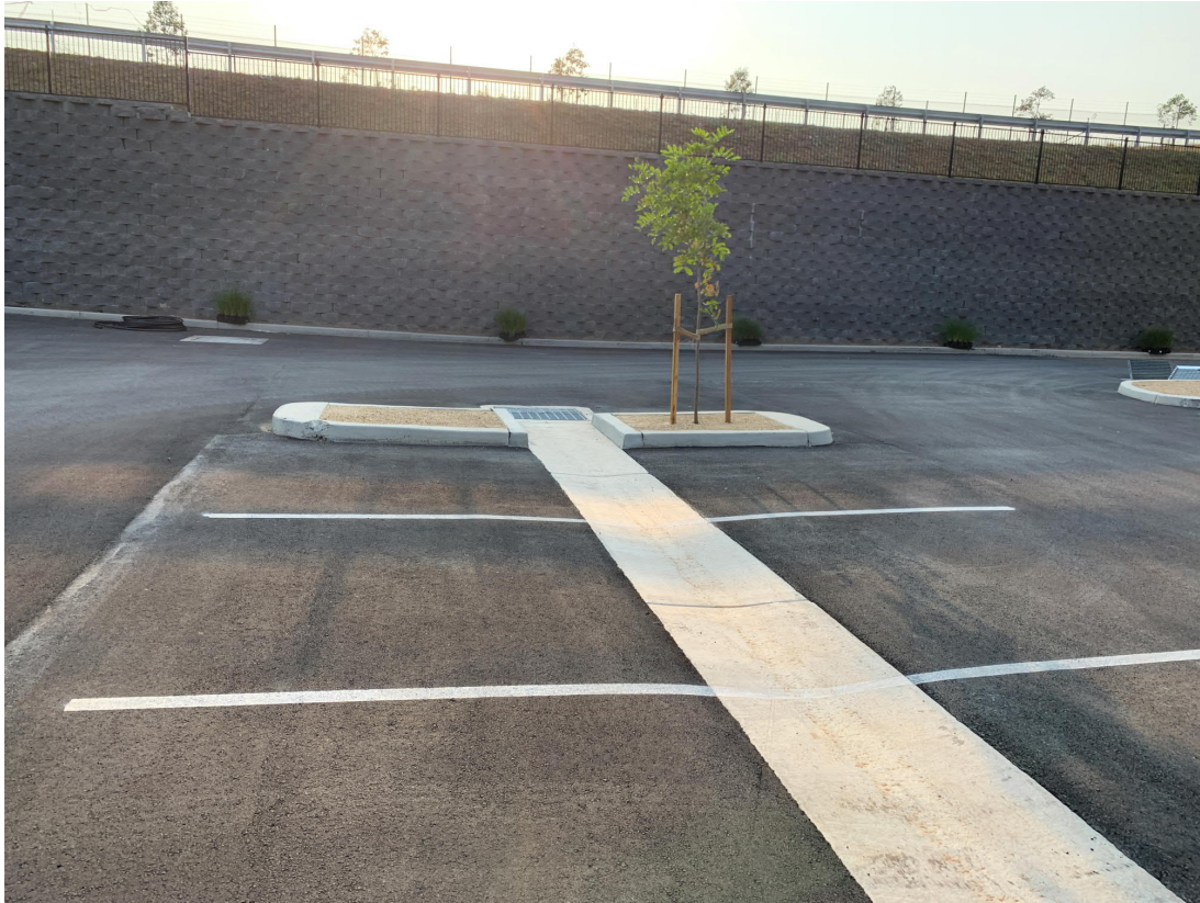
Figure 7: Example of retaining wall in location of cut
