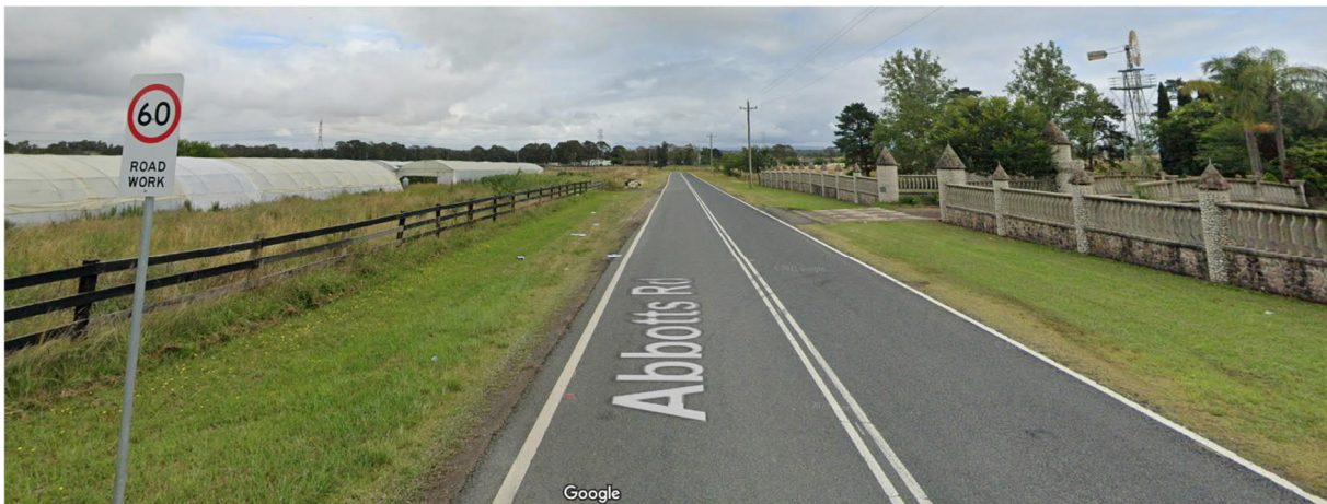
Figure 10: View of Abbotts Road looking west from Aldington Road (Google Streetview, December 2020)
