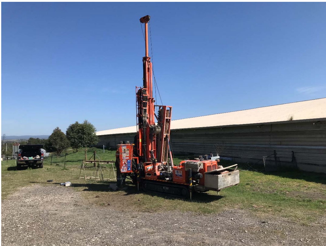
Figure 2 – Drilling rig setup in the location of BH4
