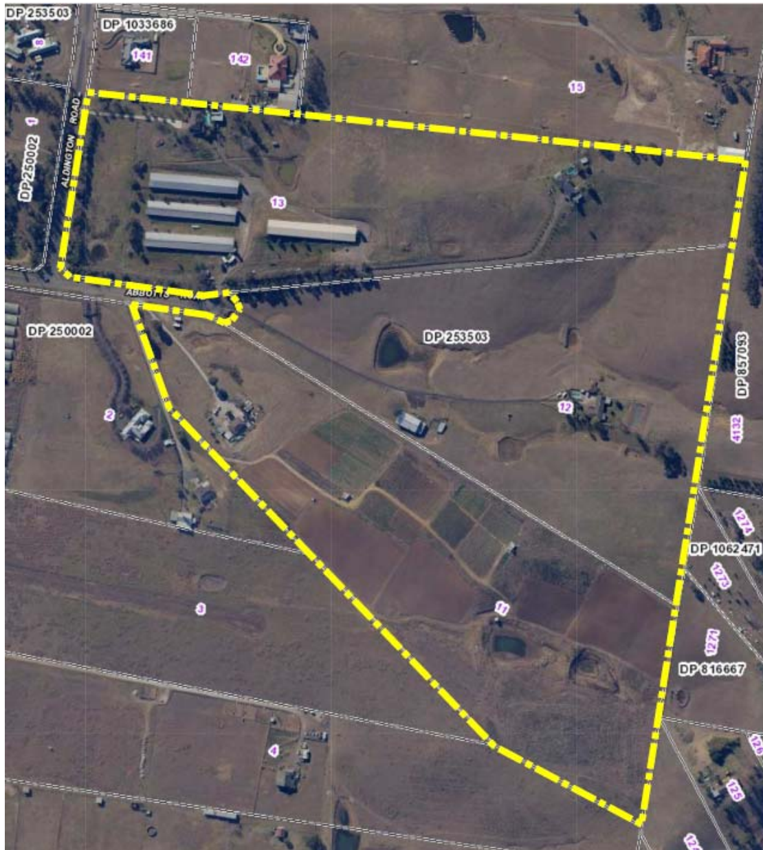
Figure 5 – Aerial Photograph of the Westlink Logistics Park Site showing adjoining landuse
