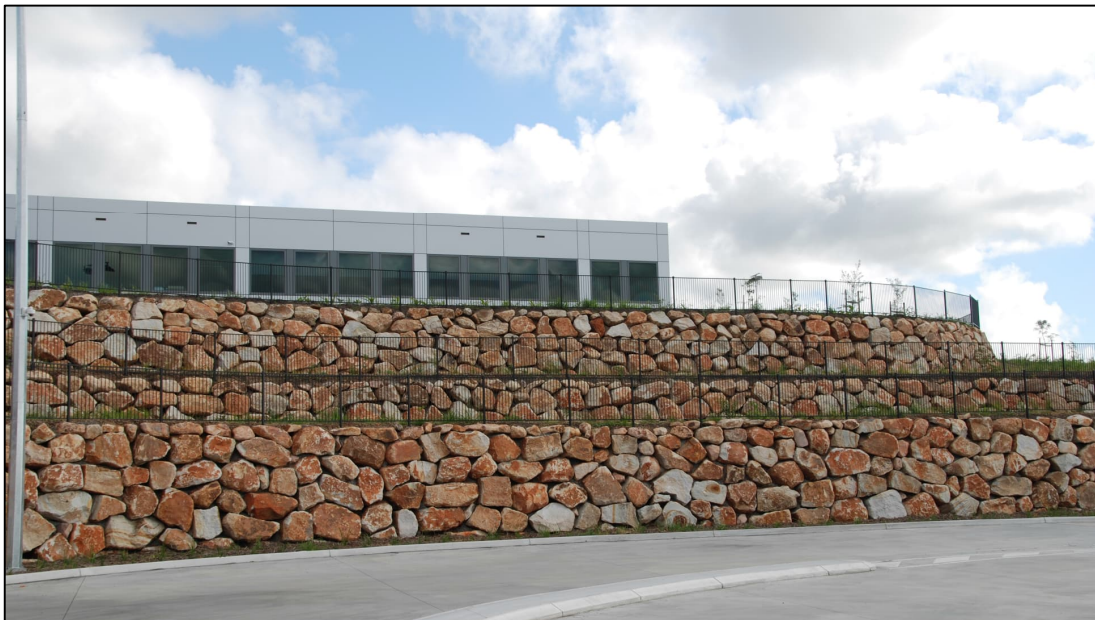
Figure 9: Tiered boulder retaining wall
