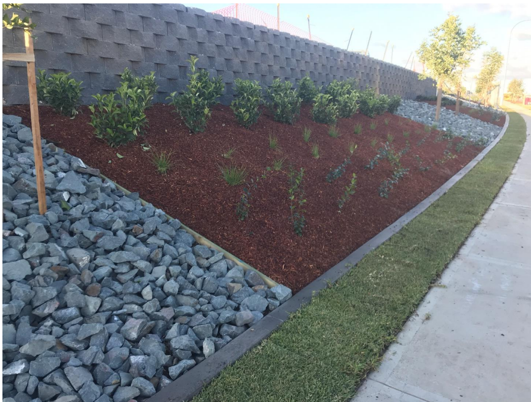
Figure 6: Example of retaining wall in location of fill adjacent to road reserve
