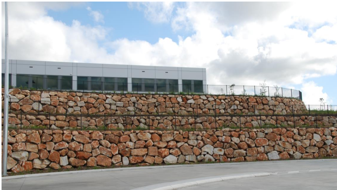
Figure 8: Tiered boulder retaining wall
