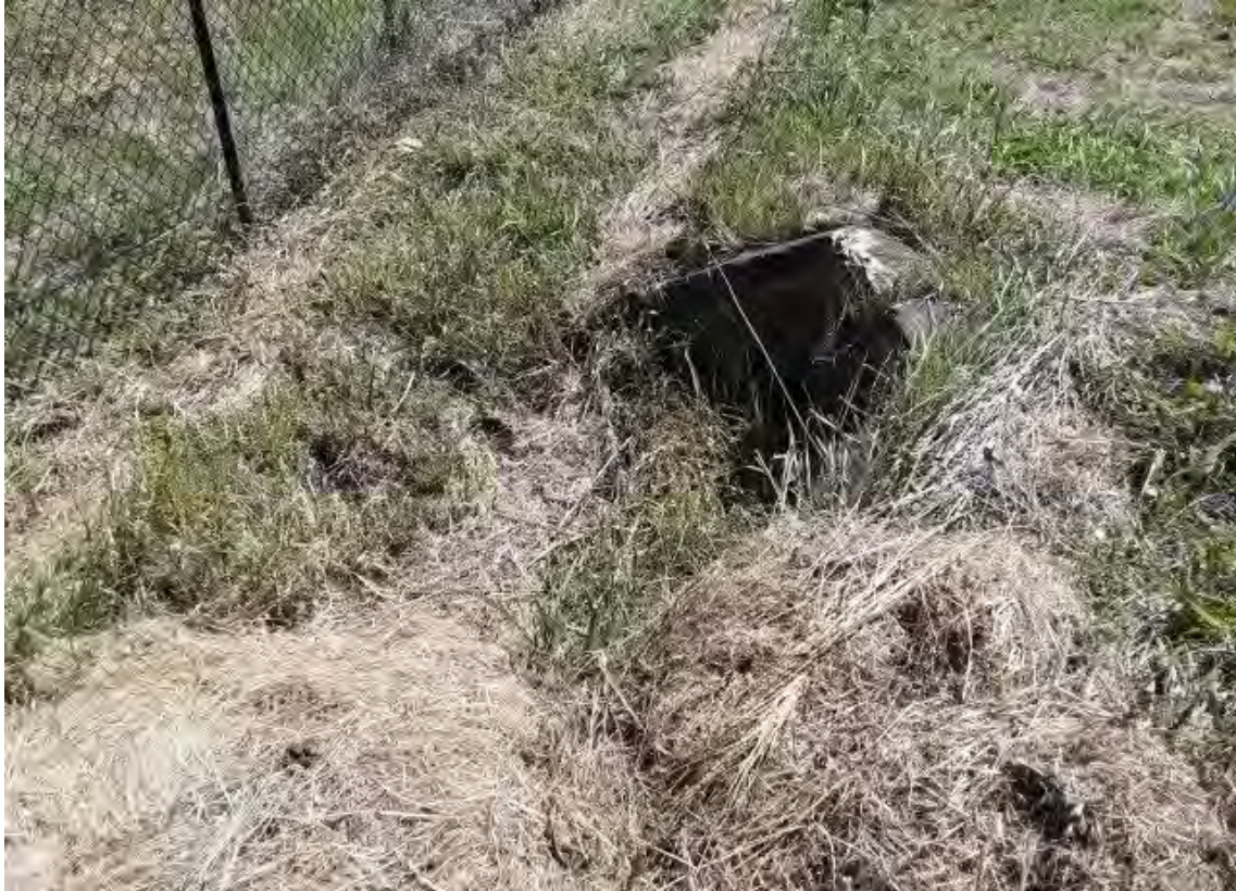
Photo 19 Area of disturbance associated with drainage
