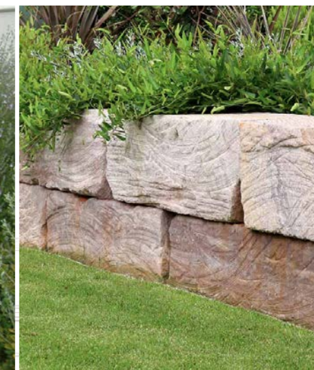
Sandstone log retaining walls
