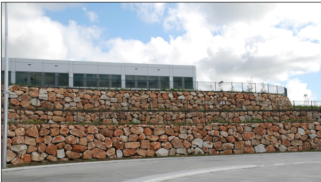
Figure 9: Tiered boulder retaining wall
