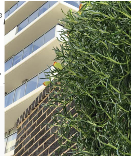
Cascading planting down retaining walls
