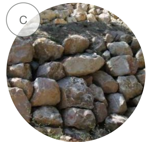
Sandstone rip rap wall
