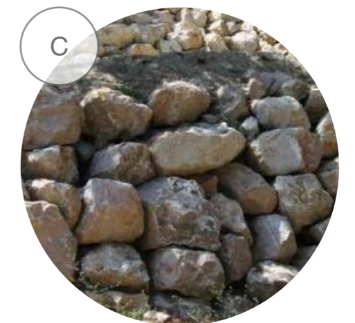
Sandstone rip rap wall
