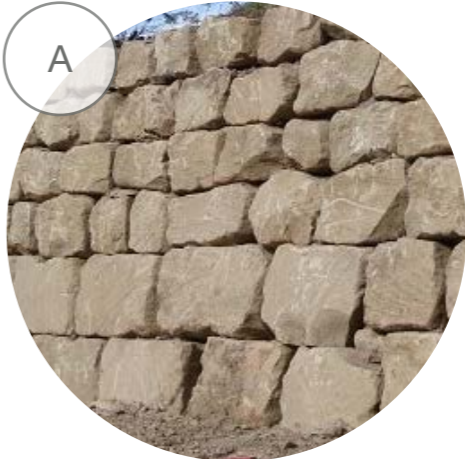
Sandstone log wall
