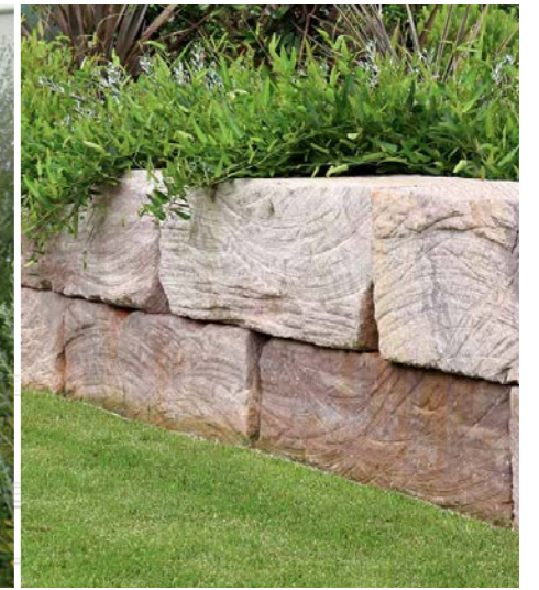
Sandstone log retaining walls
