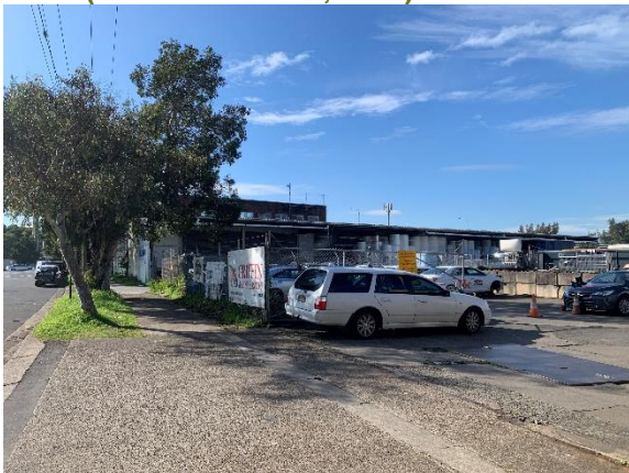
Figure 19. Eastward view to no.30 from Burrows Road (Source: Artefact, 2022)
