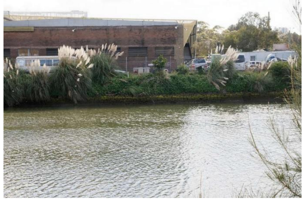
Figure 65. Alexandra Canal wall adjacent to 30 Burrows Road (Source: LOGOS, 2022)
