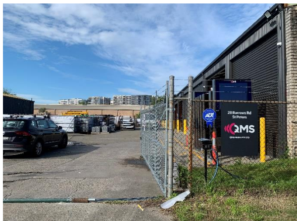
Figure 35. View of entry, looking south from Burrows Road (Source: Artefact, 2022)
