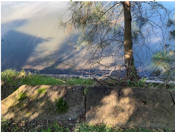
Figure 60. Sandstone capstone of Alexandra Canal Sandstone wall (Source: Artefact, 2022)
