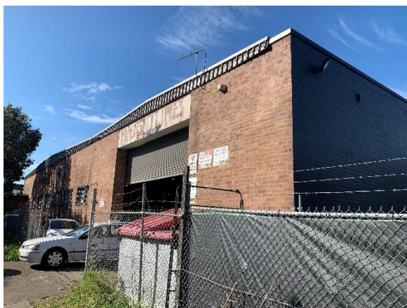
Figure 13. Western extent of no.30, looking eastwards from Burrows Road (Source: Artefact, 2022)
