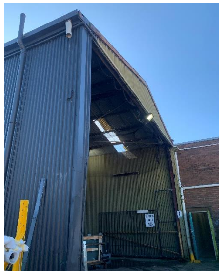
Figure 57. Exterior of shed (Source: Artefact, 2022)
