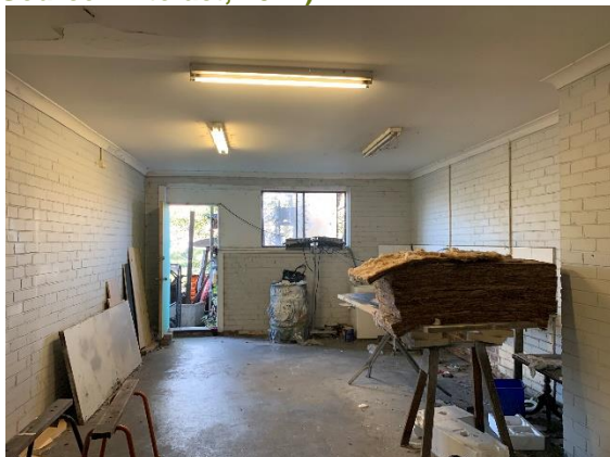
Figure 31. Interior of south-western room, accessible from southern façade. (Source: Artefact, 2022)
