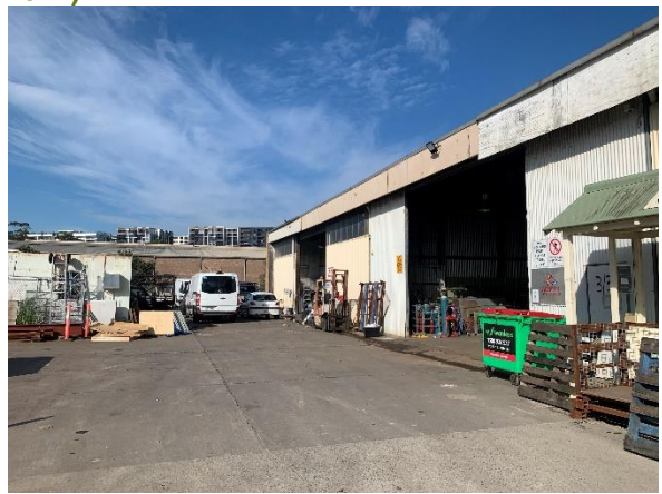
Figure 24. Southern extent of the warehouse building, looking south-west from the car park (Source: Artefact, 2022)
