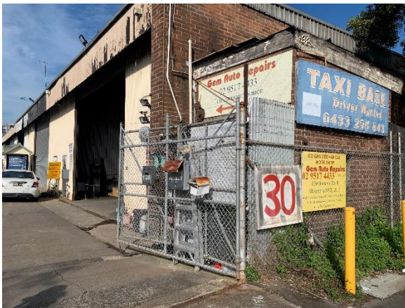
Figure 17. Intersection between northern and eastern facades, looking south from Burrows Road (Source: Artefact, 2022)
