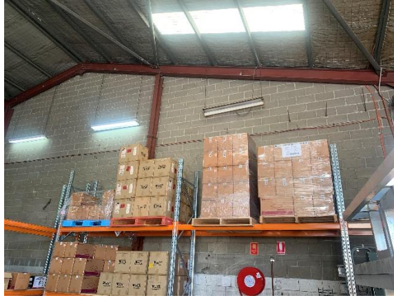
Figure 43. Interior of northernmost extent of shed (Source: Artefact, 2022)
