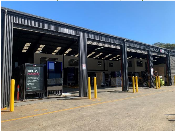
Figure 40. Detail of eastern façade. Metal sheeting appears new. (Source: Artefact, 2022)
