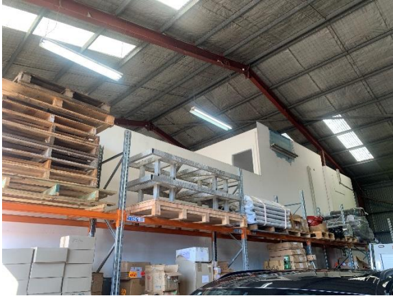
Figure 42. Interior of northernmost extent of shed (Source: Artefact, 2022)
