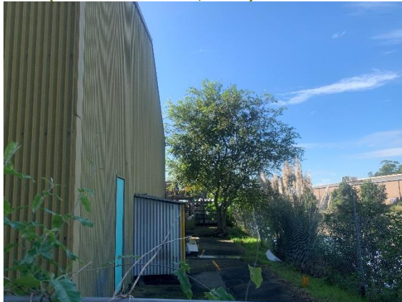
Figure 46. Southern façade, looking east (Source: Artefact, 2022)
