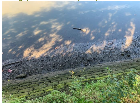
Figure 53. Detail of the Alexandra Canal wall (Source: Artefact, 2022)
