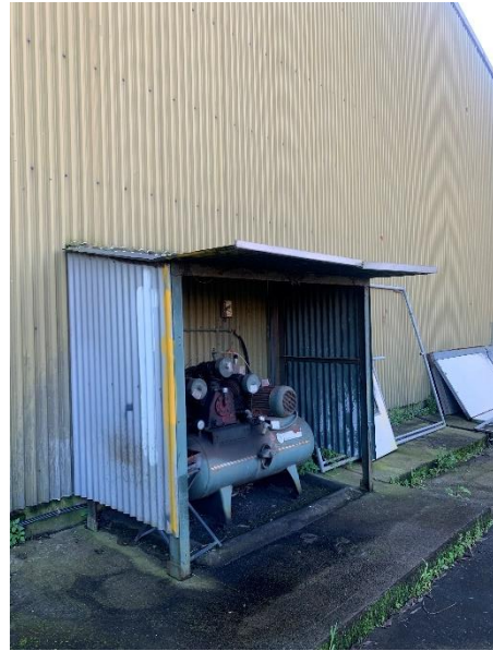
Figure 49. Detail of machinery and awning to southern façade (Source: Artefact, 2022)
