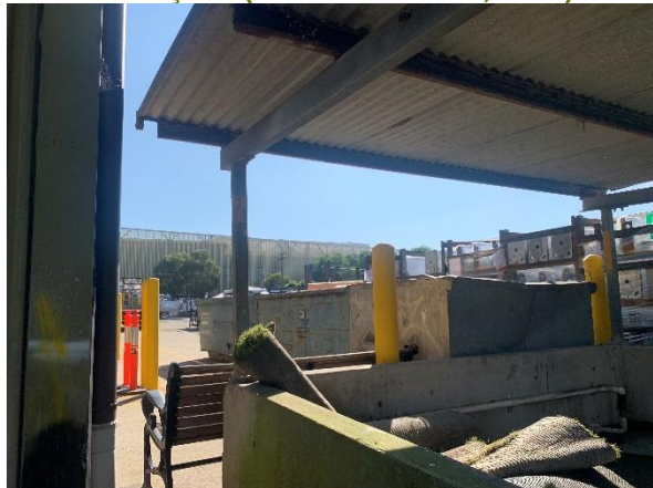
Figure 51. Detail of concrete structure with awning. (Source: Artefact, 2022)
