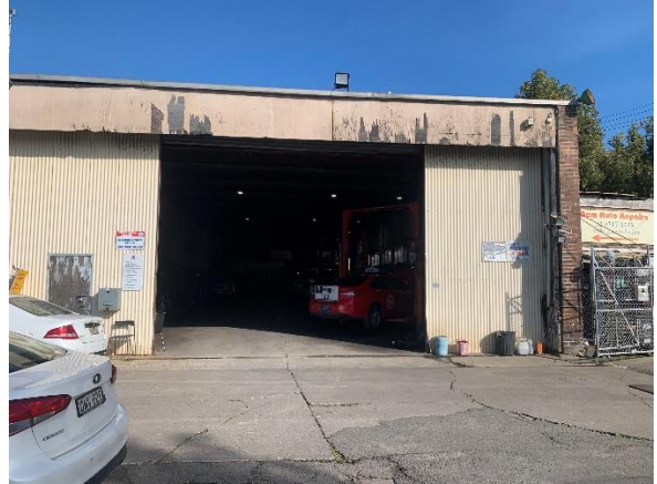
Figure 22. Looking west towards the eastern façade of the warehouse (Source: Artefact, 2022)
