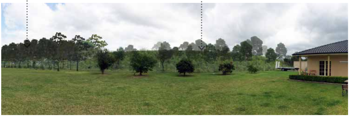
Representation of reconstructed bund, with supplementary planting preventing views into the site
