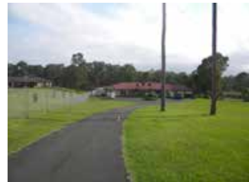
3 - View point looking north from driveway
