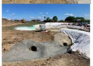
It was suggested that the dosing unit be moved to the upper pipe or to a 3<sup>rd</sup> inlet pipe within the channel so that the doing does not need to be shared between two active inlets.
