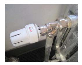
Thermostatic Radiator Valve (TRV)
