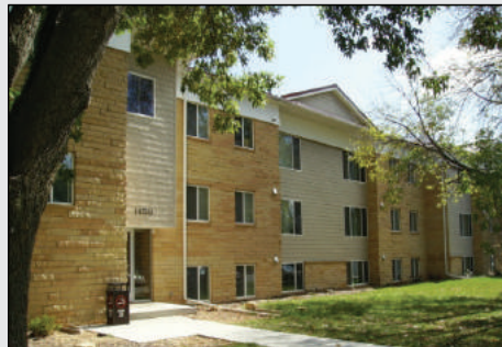
Viking Terrace; Energy Efficient and Healthy Housing in Worthington, MN
