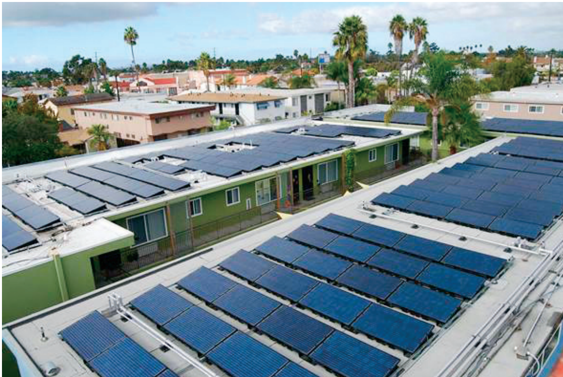
A 58-kilowatt solar photovoltaic (PV) system atop the 34-unit Townspeople Apartments in San Diego.
