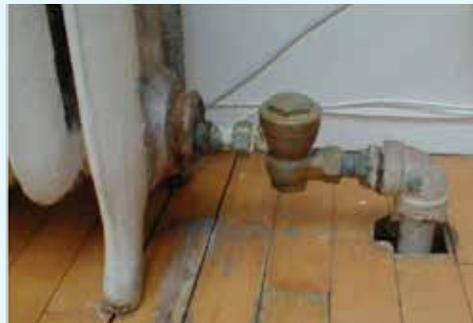
Figure 5: In-Unit Steam Trap
