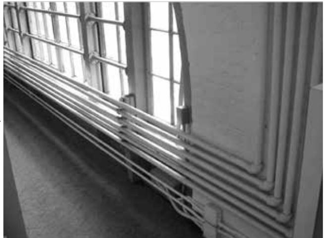
Figure 23: Hydronic System Piping
