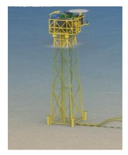
Figure 4.18: Typical Wellhead Platform
