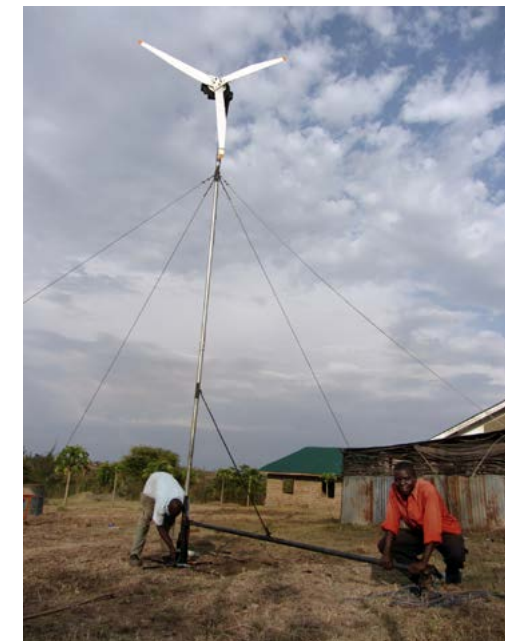
Installing a home-made wind turbine at a clinic in Homa Bay county.
