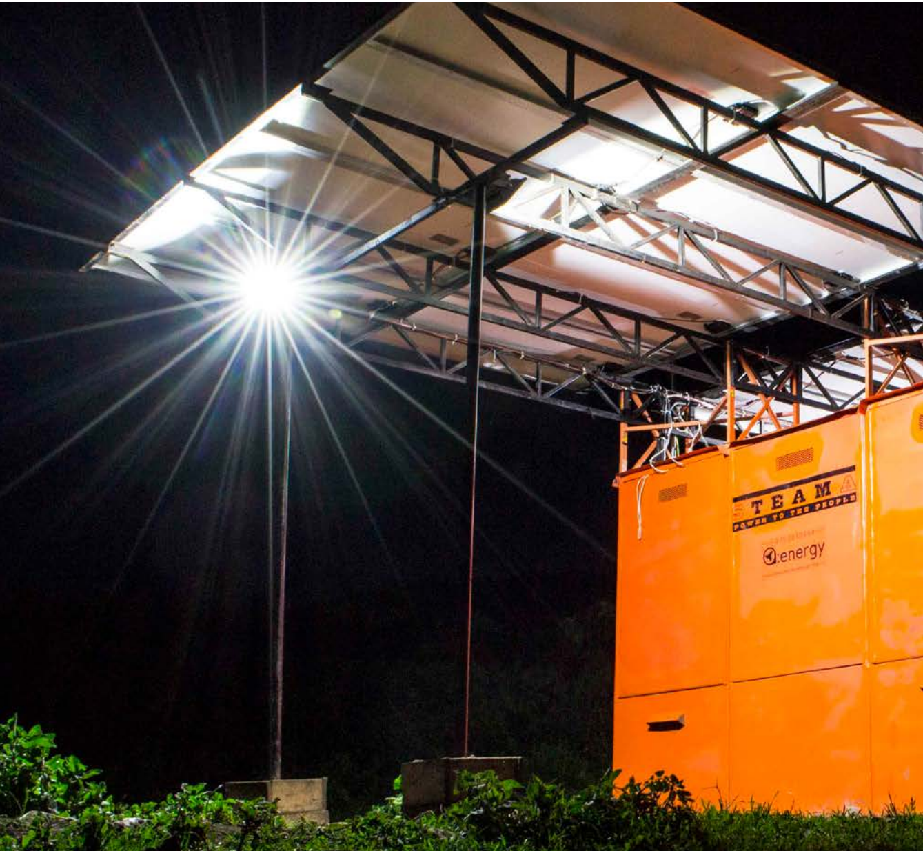
Although security lights such as these on a Power Hub at Olturoto definitely help, bringing tangible value to a community seems to be the best security of all.
